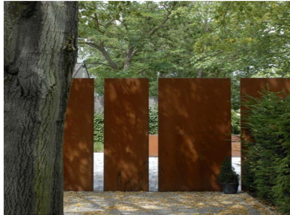
The fence around the hospital in Harrogate, North Yorkshire, England. Brand S355K2W + N
