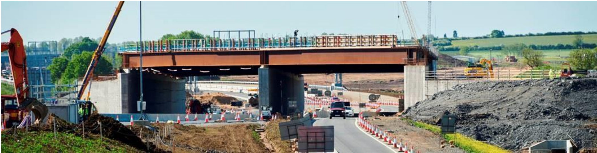
Project Cleveland Bridge, UK, capacity 3700 tons, steel grade S355J2W + N
