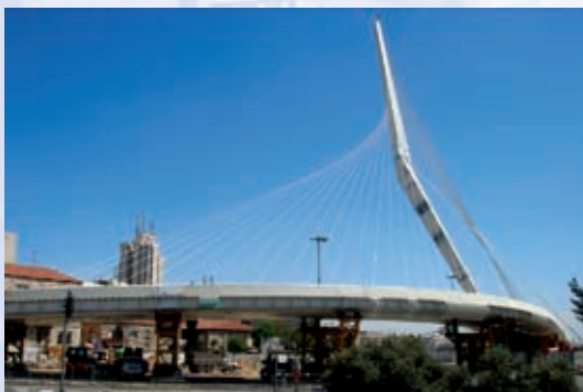
Bridge for the Light Rail project Jerusalem, Israel Cable-stayed structures (locked-coil wire ropes, caps)
