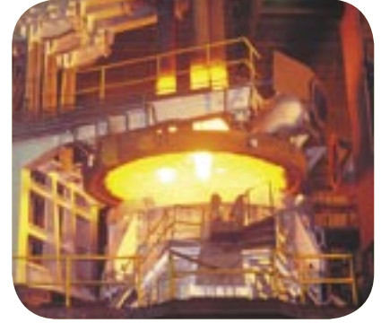
Electric Arc Furnace
