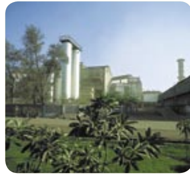
State-of-the-art Fume Extraction System at Hot Rolling Division.
