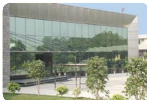
Tulsi Bhawan, the R&D Complex at Hisar, India
