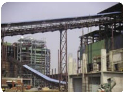
Work in Progress, at the Greenfield Project
