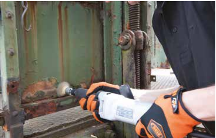
Paint and rust removal by using end brushes with crimped wire bristles on a straight grinder
