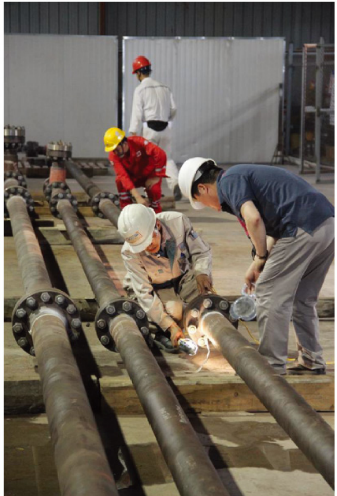
Separated from control room
